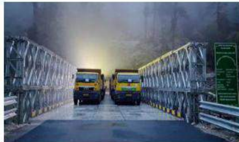
Double Lane Modular Steel Bridge
