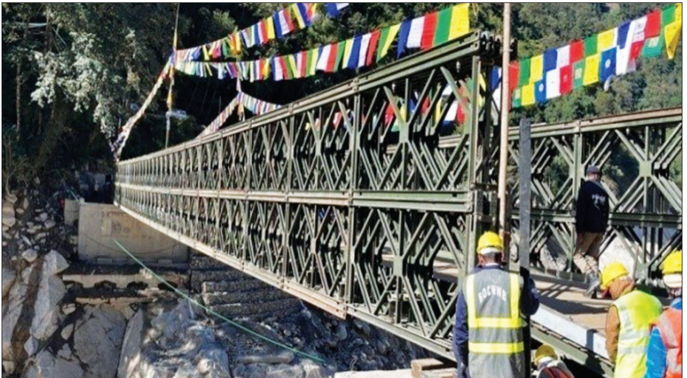
Chungthang Bridge Launched on Nov 15, 2023
