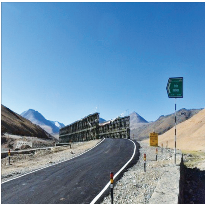
Demchok in UT of Ladakh
