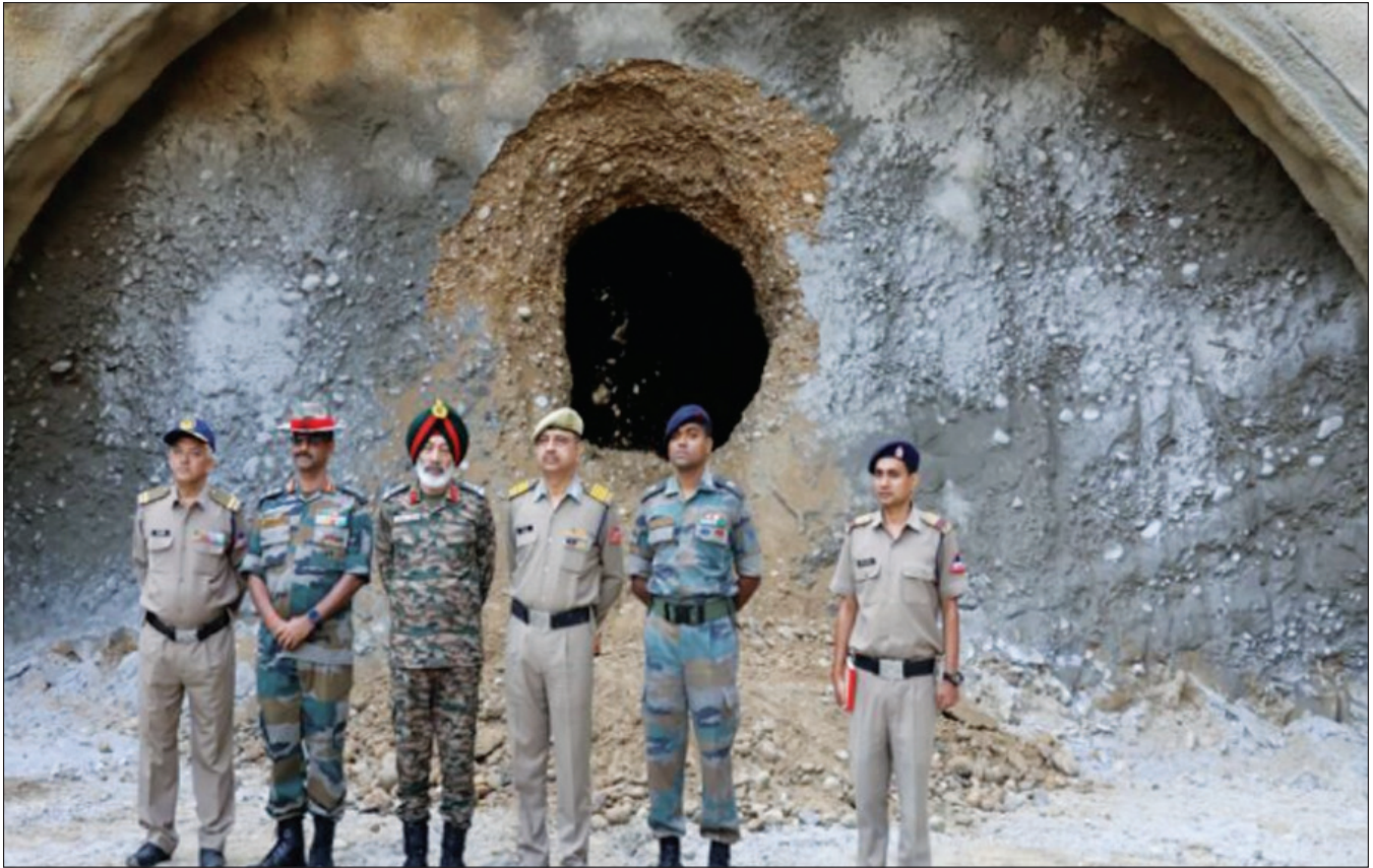
Breakthrough on Kandi Tunnel on Road Akhnoor-Poonch on Oct 25, 2023
