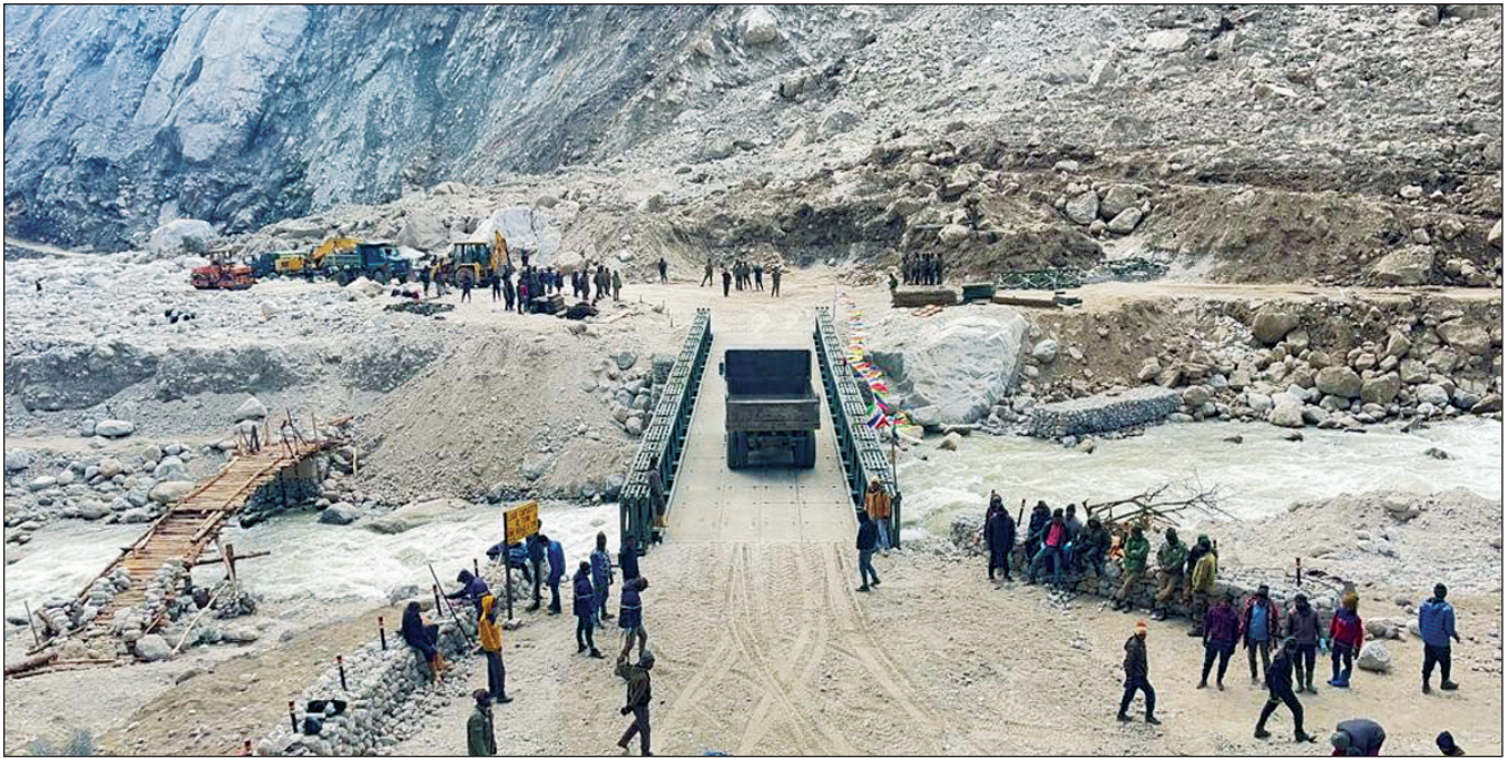
Zeema Bridge Launched on Nov 28, 2023
